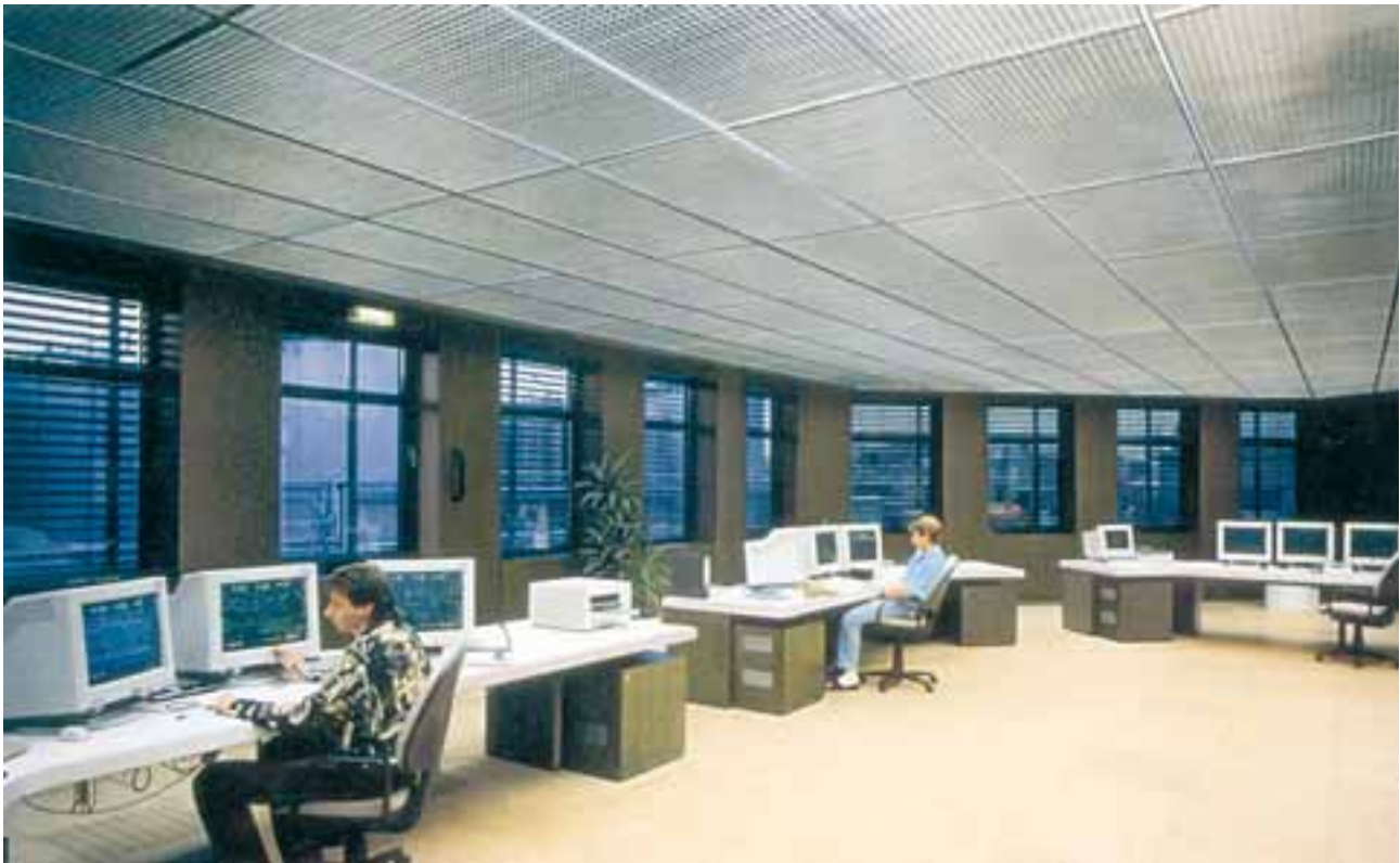
Control room of a refinery
